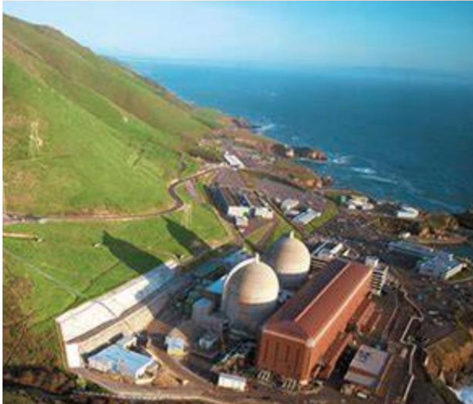
The Diablo Canyon Power Plant provides about 9% of California's power needs
